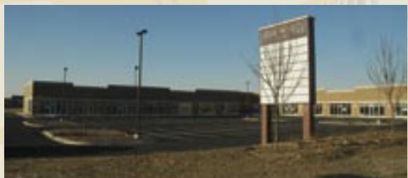
Fox Hill Center, located at the southwest corner of Rt. 34 and Sycamore Road, offers 24,000 square feet of retail/office space configured in 1,258-square-foot and larger units. For more information, call Les Kristof at 630.572.5607.
