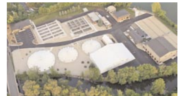
An overhead view of the Yorkville-Bristol Sanitary District located at 304 River Street
