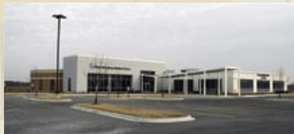
Dreyer Medical Clinic and Provena-Mercy has opened its 22,000-square-foot state-of-the-art medical office building on Route 34 near Sycamore St.
