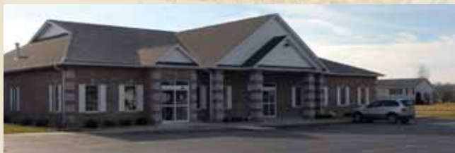
The 8,000-square-foot new Valley West Medical Arts Building is located at Countryside and Center Parkways. This building is a joint venture of Yorkville MRI, which offers diagnostic imaging services, and Valley West Community Hospital, which is leasing space for physicians' offices. For information, call 815-756-1521, ext. 3660.
