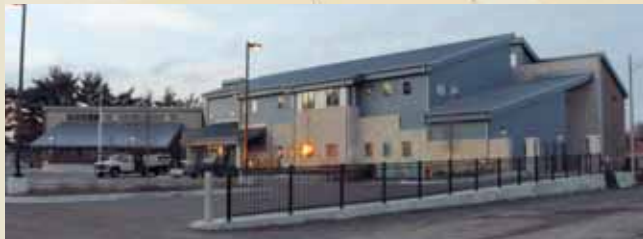
The new 34,000-square-foot addition to the Yorkville Public Library opens in February adjoining the original 6,000-square-foot building at 902 Game Farm Rd. The new facility includes a Children's Library, a Children's Program Room, a Young Adult Area, and an Adult Quiet Reading Room. Call 630-553-4353 for more information.
